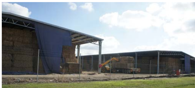
Hay shed at the Wingara facility in Epsom, Bendigo.
